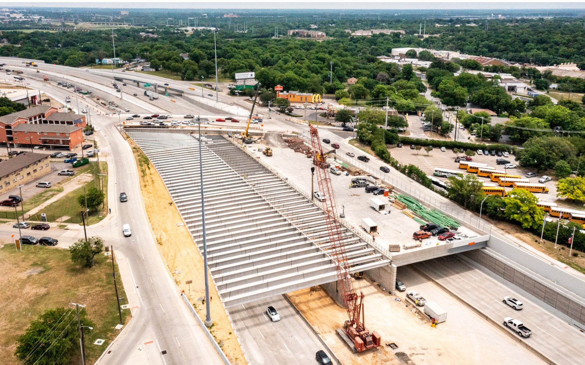
Construction crews begin capping Interstate 35 to make new ground for Halperin Park in Dallas, TX. Photo: David Lloyd / SWA
