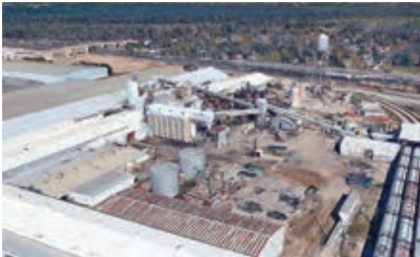
EXISTING INDUSTRIAL CONDITION
