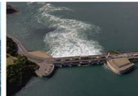
Tidal Power Plant_ la rance, France
