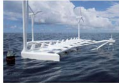
FLOATING POWER PLANT_Denmark
