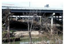
Above: Existing conditions of the downtown section of Buffalo Bayou in the mid-to-late 1990s. This photo documents the impact of seasonal storm flows within the bayou's fluvial and coastal mud flat marsh origins. Visually, the eroding clay, silt, and fine-sand banks are devoid of riparian plant growth that would have normally protected the banks.
