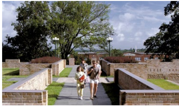
+ Sam Houston State University, Old Main Restoration Huntsville, Texas
