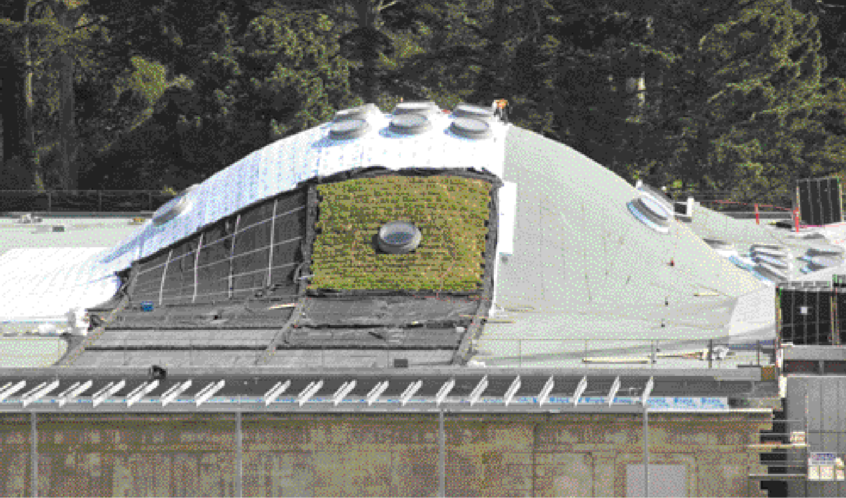
Several layers of the soil structure are visible in this picture. Testing continued throughout construction to determine the best planting solutions. Here a section of turf is being used to test the stability of the soil system.
