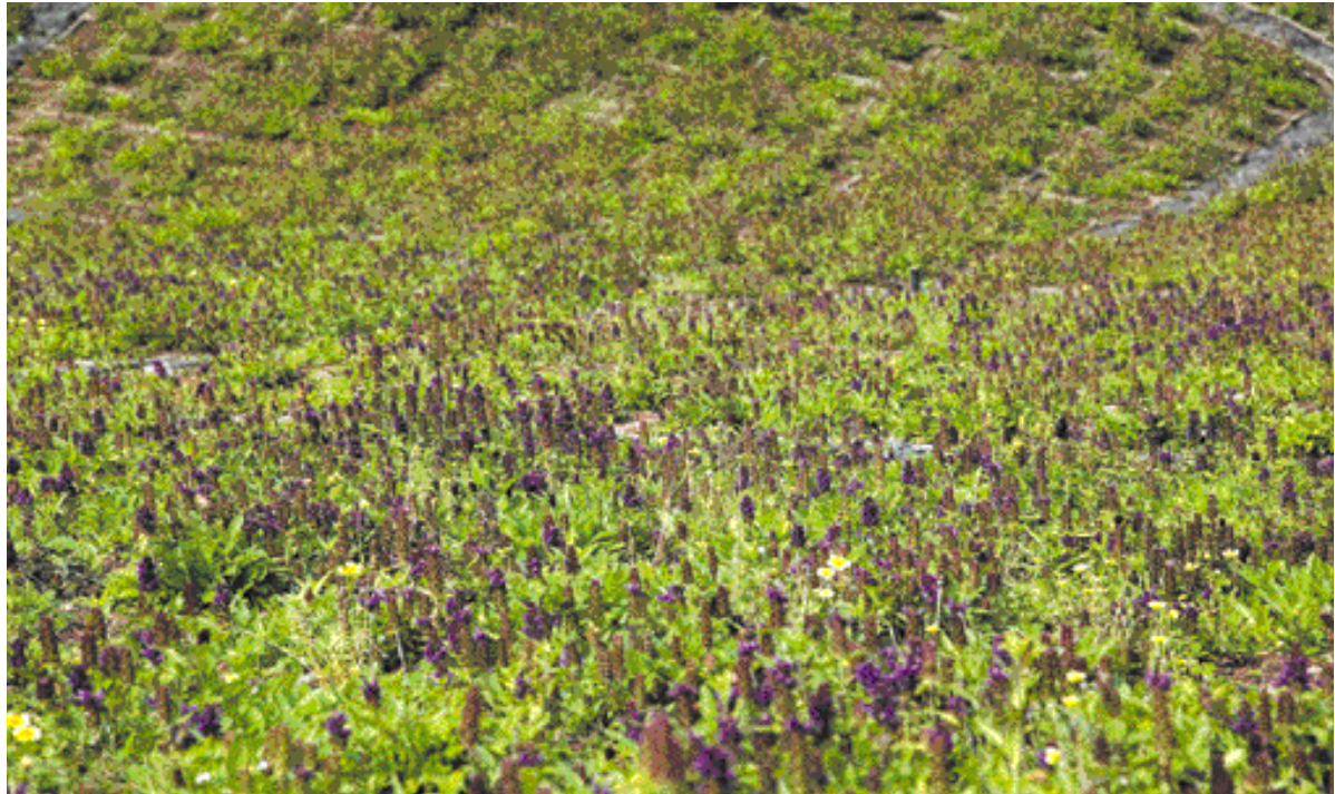
The roof will consist of California selected native plant material suited because adapted to San Francisco's highly seasonal natural irrigation patterns. All draining storm water runoff is directed back into the water table.
